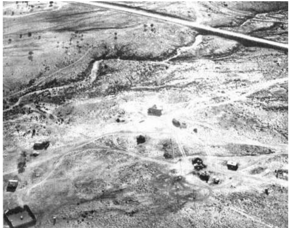
Yazzi Camp, an extended family settlement. The rectangular one- to three-room houses are occupied by members of several families interrelated by common blood lines and marriage. The symmetrically rounded buildings are hogwaddies, traditional Navajo houses. Sheep corrals and stacks of firewood suggest a subsistence mode of life support. The utility poles carry telephone service into the encampment. Radiating patterns of roads are common to most clusters of the dispersed dwellings in Navajo country.
